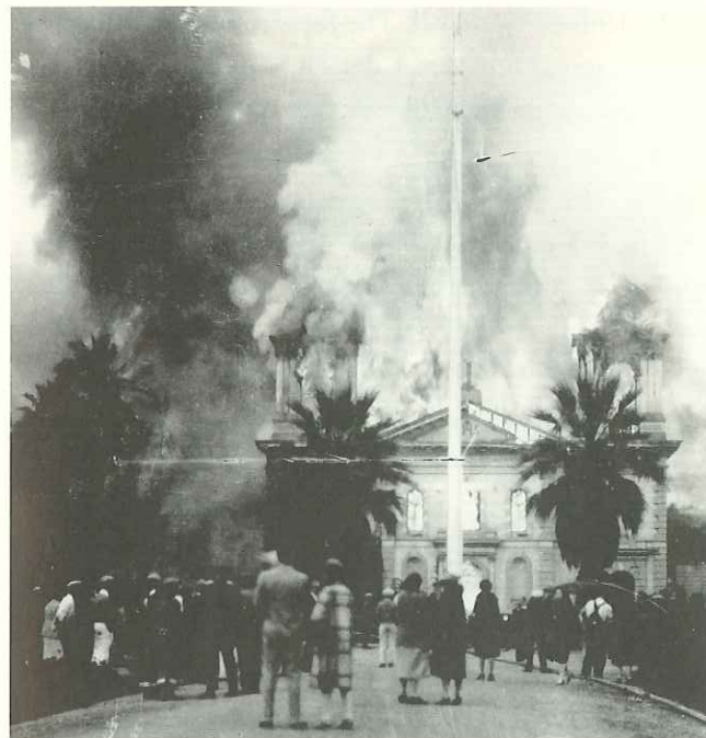
The Mission Church was destroyed by fire in 1926.
