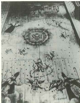
The Mexican artist Agustín Dávila, with the help of Native American assistants, painted this sanctuary ceiling on redwood slabs in 1824–25. Both the reredos and the ceiling were destroyed in the fire of 1926.
