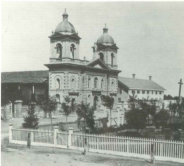
The façade of the Mission Church as remodeled in 1861 by President Villiger.
